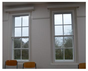
All of Selectaglaze's units are tailor made to ensure the tightest fit and use twin seals to virtually eliminate draughts and reducing heat loss by up to 50%. Secondary glazing can also reduce noise ingress creating a quieter environment and a reduction of 45dB is easily achievable.
