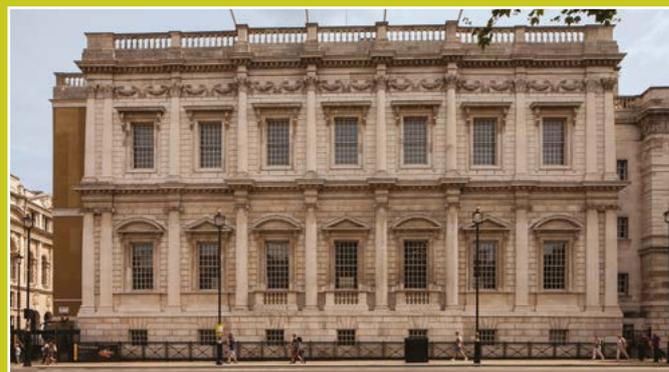
Selectaglaze has products certified to the requirement, but they had never been specified to these sizes (the Main Hall window openings were 3.6m high and 2.0m wide). Blast testing was carried out on the largest ever single casement to be tested in the UK. The results were a success and planning for the installation began.
