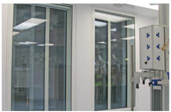
The wards provided a particular challenge as it was essential they remain fully functional at all times. To resolve problems associated with masonry drilling Selectaglaze and Skanska devised a system of wedging and bonding timber sub frames into the window reveals which supported slimline fixed glazed panels.
