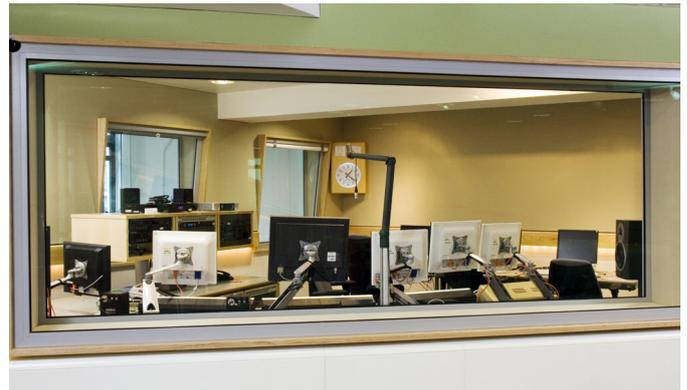
angled at 5 degrees and glazed with 10.8mm Amiran anti-reflective Optiwhite acoustic laminate glass from Schott. The largest of these panels being almost 3 metres long.
