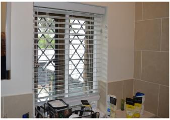
The inclusion of a low emissivity hard coat on the laminate glass reduces the U-value of the window combination to the range 1.7 to 1.9 W/m2K.
