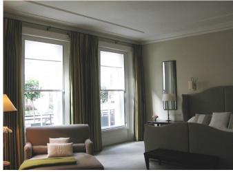
The windows were specified with laminated glass to provide high noise insulation levels and additional safety. Sound tests conducted at the Taywood Laboratory demonstrate that Selectaglaze systems can achieve 45dB sound reduction and so ensure a quiet and peaceful environment, even in busy city centres.
