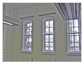
Secondary glazing, not to be confused with doubleglazing, involves the installation of an additional internal window. In addition to noise insulation, secondary glazing will improve energy efficiency and provide increased security. The product is particularly appropriate for exam rooms, music rooms, computer labs and secure reception areas.
