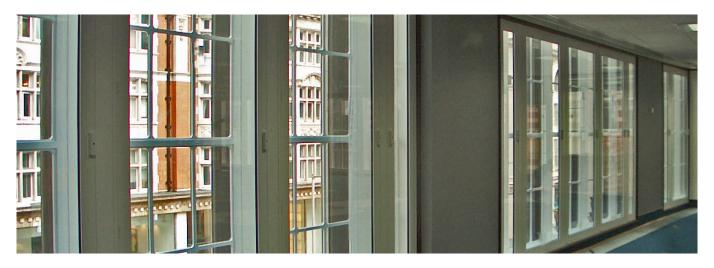
A 200mm gap between the original steel windows and the secondary installation ensured the most effective noise control.
