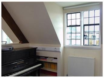
The introduction of secondary glazing immediately increases the thermal retention of a building, and on this project Selectaglaze also used a 6mm toughed low-E glass which can enhance the U-value to around 1.95.
