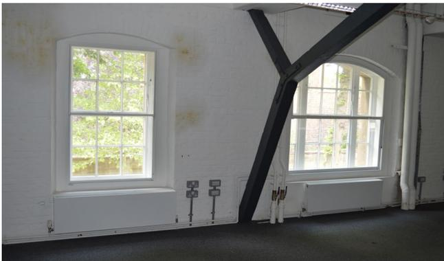
The Grade II Listed Engineering workshop, also part of the University of Kent, underwent a refurbishment in 2013. Selectaglaze was approached by main contractor Coombs Canterbury Ltd to provide secondary glazing for noise insulation and thermal retention. 21 units were installed on the ground and first floor windows including a number of Series 45 bottom hung and fixed lights, and Series 20 Vertical
