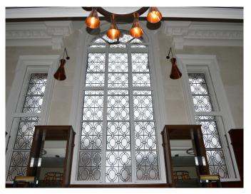
Secondary glazing is an independent window installed on the room side of a building, which reduces noise ingress creating a quieter environment and a reduction of 45dB is easily achievable. It not only effectively reduces external noise, but can also virtually eliminate draughts and aids in retaining the heat of a building, reducing heat loss by up to 50%.
