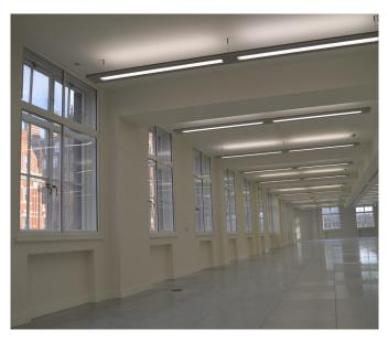
The minimal frames created clean lines complimenting existing primary windows, making them unobtrusive and virtually unnoticeable. Selectaglaze's units are a fully reversible adaptation accepted by most heritage bodies.
