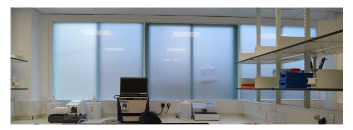
Selectaglaze met the brief by installing a total of 15 horizontal slider units with 6mm toughened low-E glass in the 2 and 3 pane options to all of the external primary windows. The inverted u-channel section was included to sit in the bottom of each frame to minimise the dust traps and enhance the ease of cleaning. This is ideal for tissue culture labs where there is a requirement for infection control.
