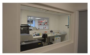
In addition, a total of 22 Series 40 fixed light units were fitted as viewing panels in the research and development laboratories. The Series 40 has a sturdier frame which can house higher weights of glass than required in a standard
