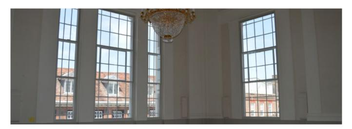
as sympathetic as possible to the original window design. It was constructed with powder painted aluminium sections to match existing paintwork and 6.8mm low emissivity laminated glass. The finished installation was inspected and approved allowing the remaining windows to be treated.
