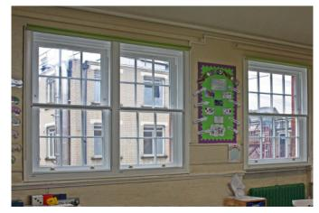
Selectaglaze treated a total of 37 windows across all four floors of the school, providing a total of 69 frames, each of which was purpose made with high performance seals that not only improves the acoustic insulation but also helps reduce the passage of dust and dirt, which is a feature of all building sites.
