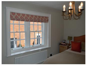
single glazed primary windows throughout. Additionally, the other requirement was noise insulation from the busy thoroughfare. Due to the Listed status of the building, these windows could not be replaced. Osprey Developments consulted Selectaglaze, the leading specialist of secondary glazing for a solution.
