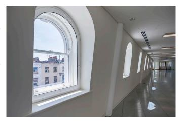
When there is a cavity of at least 100mm between the primary and secondary glazing a reduction of 45dB is achievable. An additional benefit of secondary glazing is thermal retention, with the use of high performance twin seals, it virtually eradicates unwanted drafts and a U-value of 1.8 is possible.
