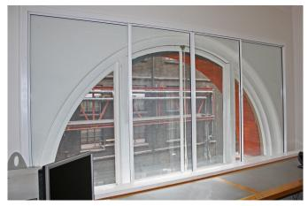
The study concluded that, prior to commencement of these works, it was essential to install acoustic secondary glazing to affected windows in order to provide acceptable working conditions in the offices.
