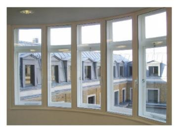
Secondary glazing systems are purpose made and arrive fully assembled to allow rapid installation with minimal disruption. They need very little maintenance and will continuously contribute to energy savings.
