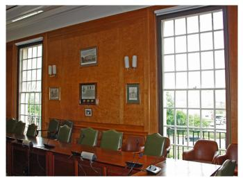
More than 270 bespoke frames were fully fabricated off-site allowing rapid installation to all four floors in phases to suit the contractors programme. The result is a more energy efficient and comfortable environment that is also much quieter.
