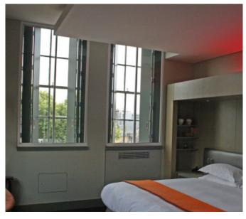
The hotel had retained the building's original sash windows and installed bi-folding shutters to the room side of the bedrooms but this combination did not provide the required level of noise insulation.
